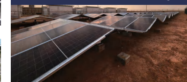
Saudi Arabia Oilfield Project
